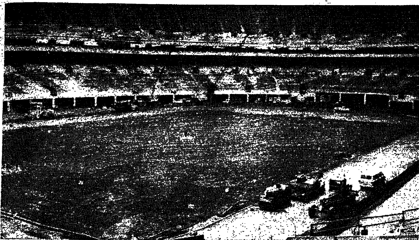
This is how the Olympic Stadium in Montreal looked Friday. To finish construction in time, there are 2,000 workers by day and 1,500 by night.
